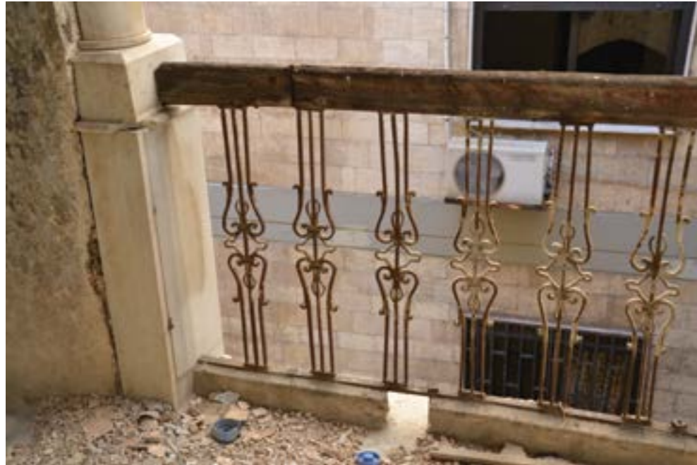
Figure 138 Metal Handrails on the balcony were detailed and designed authentically
