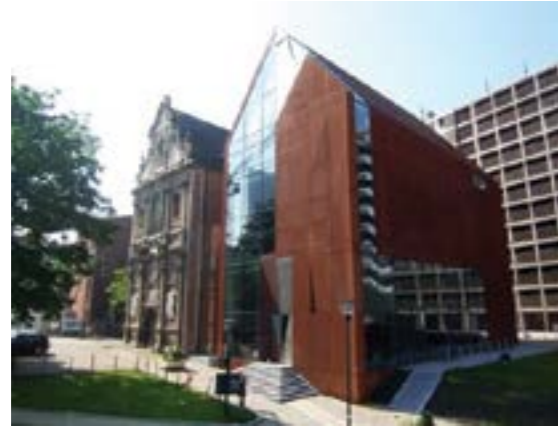
Extension des Briggittines SumProject & Studio Andrea Bruno Wallonie-Bruxelles Architectures - 2001-2005
