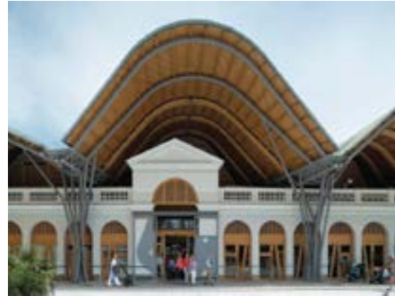
Santa Caterina Market in Barcelona, Designed by Enric Miralles & Benedetta Tagliabue Architects - 1997 - 2004
